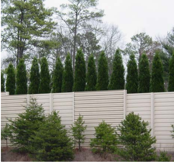
Standard steel barrier with landscaping GA 400 - Atlanta, GA (Highway view)
